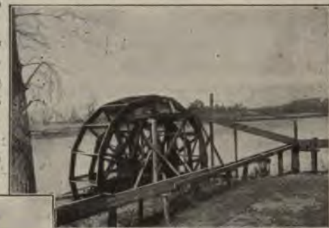
Irrigation. Sometimes a reservoir to hold water for irrigation is made by building a dam across a stream. Sometimes the water has to be pumped into a reservoir or into a flume, as shown in this view at Elgin, Utah. This water wheel runs the pump for irrigation.
